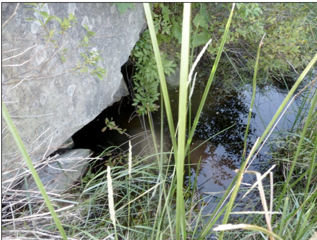
Figure 8 Culvert upstream and the undefined channel (16 September 2012).
