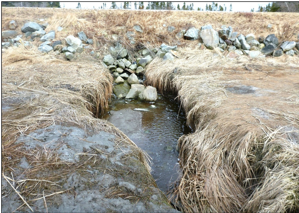
Figure 9 Downstream end of the culvert and tidal channel.
