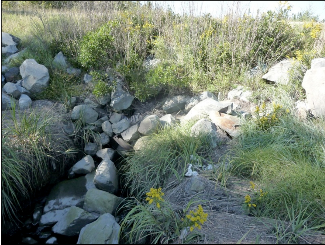
Figure 6 Downstream end of culvert (16 September 2012).
