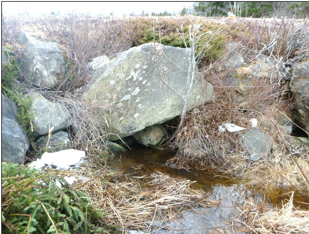
Figure 4 Upstream end of the culvert
